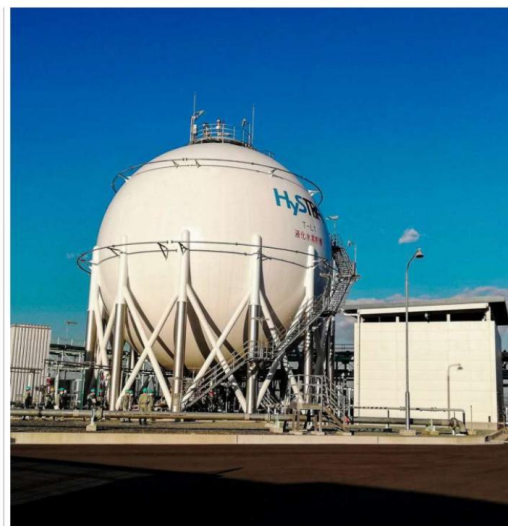
Storing for more: A 2,500 cubic-metre tank containing liquid hydrogen at Kobe Port Island plant in Kobe, Hyogo Prefecture, Japan. AP
